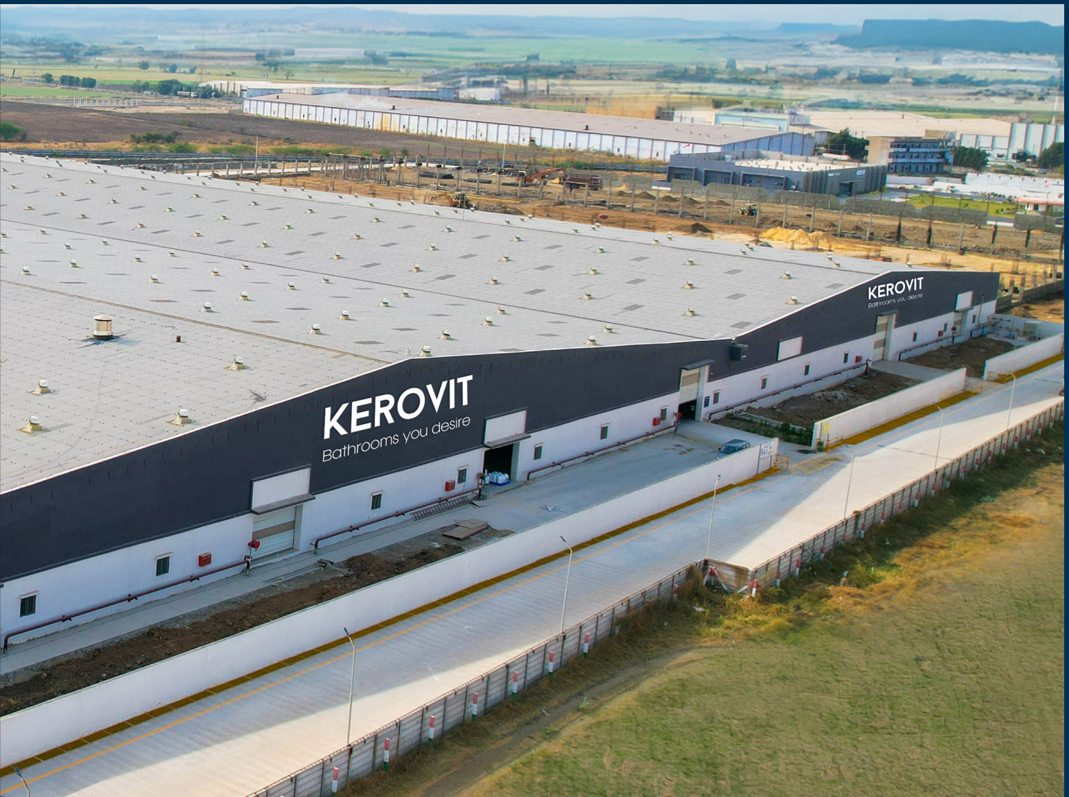
A view of KGPL Sanitaryware Plant at Morbi, Gujarat
